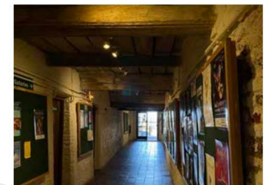
Entrance passageway from street entrance & reception to the foyer at the centre of the site
